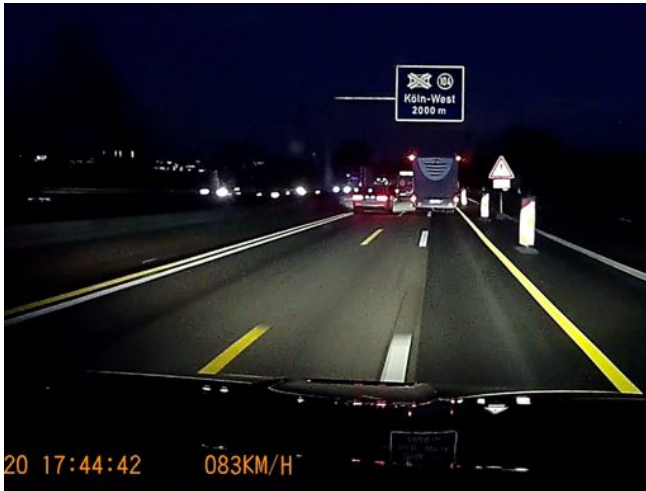
Figure 9: White lane markers are the standard ones in Germany. In construction zones yellow markers are added temporarily and overrule the white ones.
